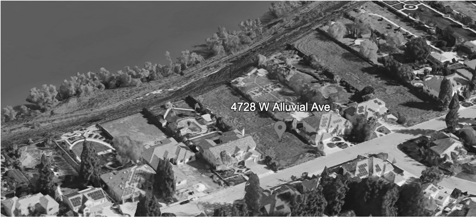
Google Earth photo | A residential grading permit was issued at 4728 W. Alluvial Ave. in Fresno.
