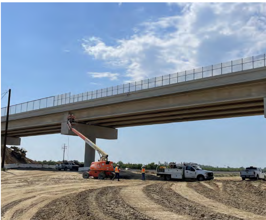
CHSRA photo | Crews work on the Floral Avenue grade separation project.
