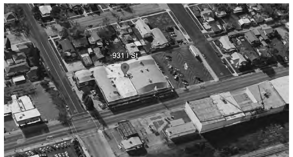
Google Earth image | An HVAC System permit was secured at 931 I St in Reedley at Valley Foods Supermarket.
