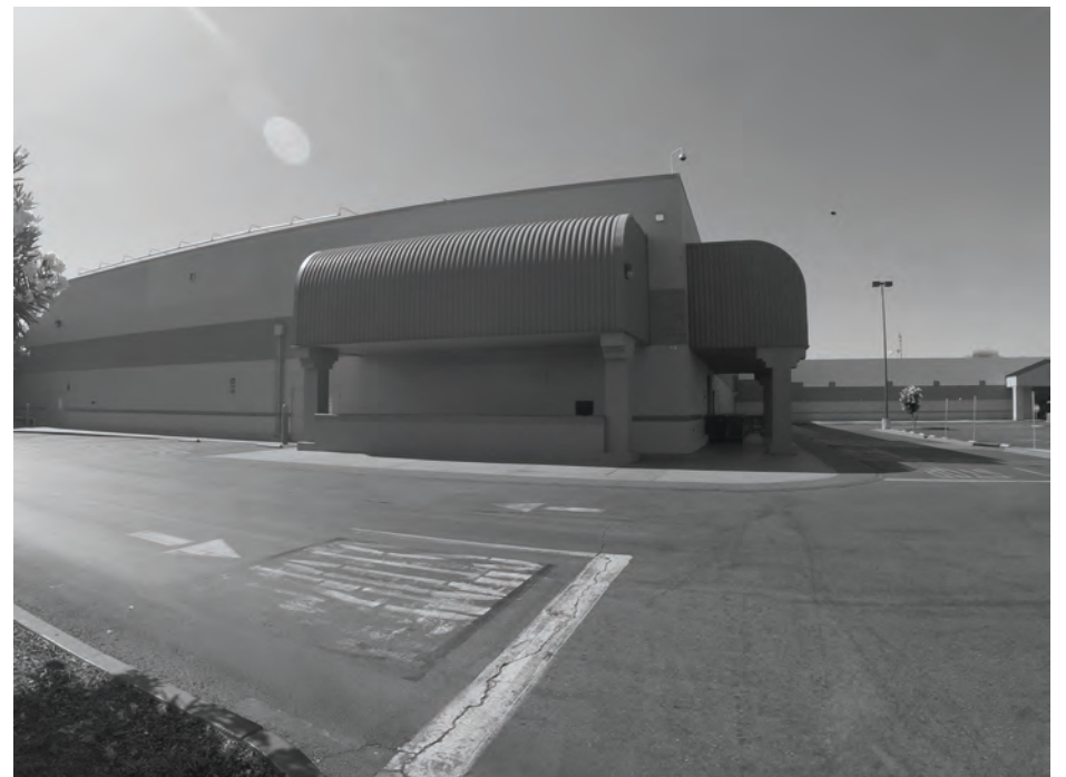
Photo by Cook Land Co. | A “before” photo shows what the former Clovis Costco looked like before improvements.
