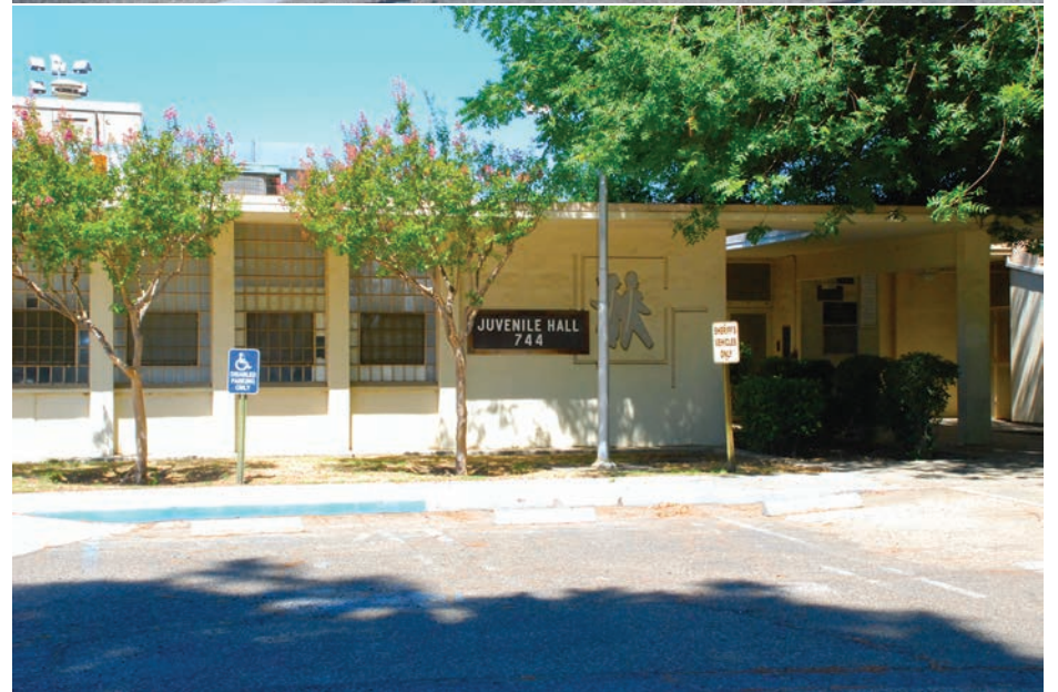
FILE PHOTOS | The Fresno Unified School District trustees may vote as soon as next week on a deal to purchase the former juvenile hall facility in Fresno, which includes several buildings on nearly 13 acres.
